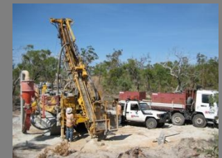
Drilling at Kingsgate
