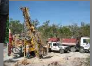
Drilling at Kingsgate
