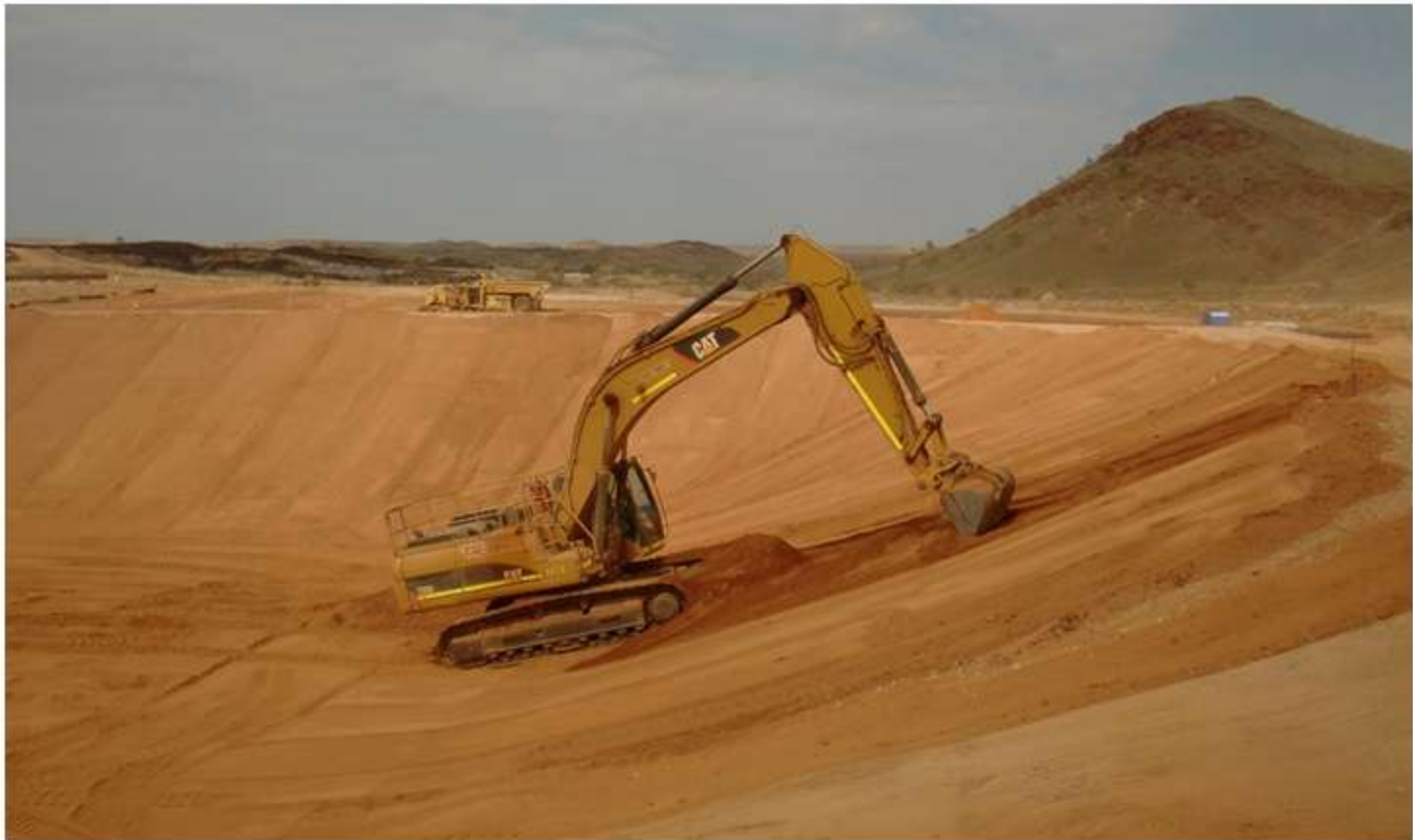
Construction Process Water Dam
