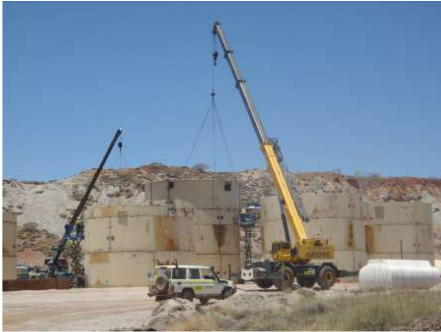
CIL tank erection in progress
