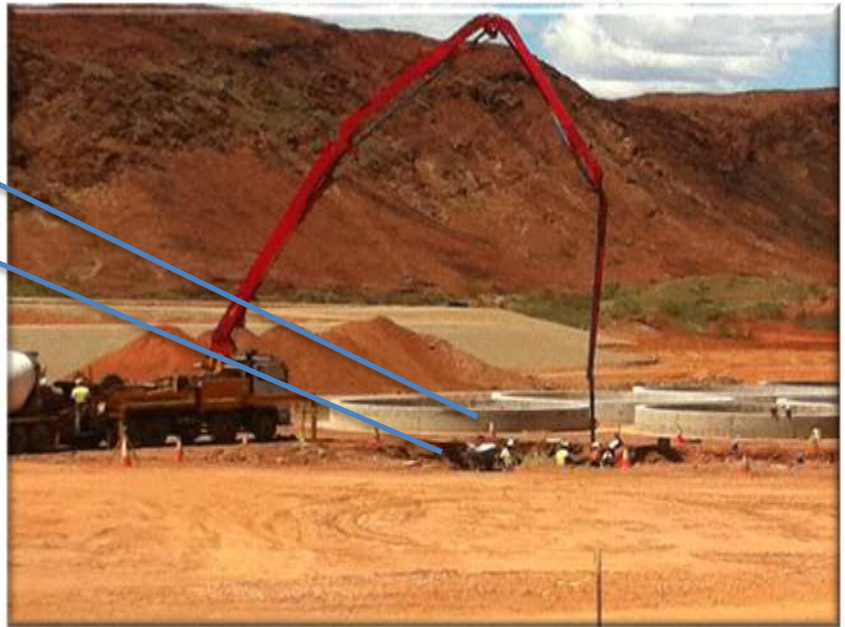
SAG Mill Foundations – pouring the blinding
