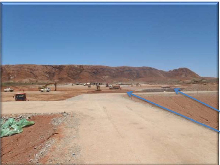
Process Plant site looking west
